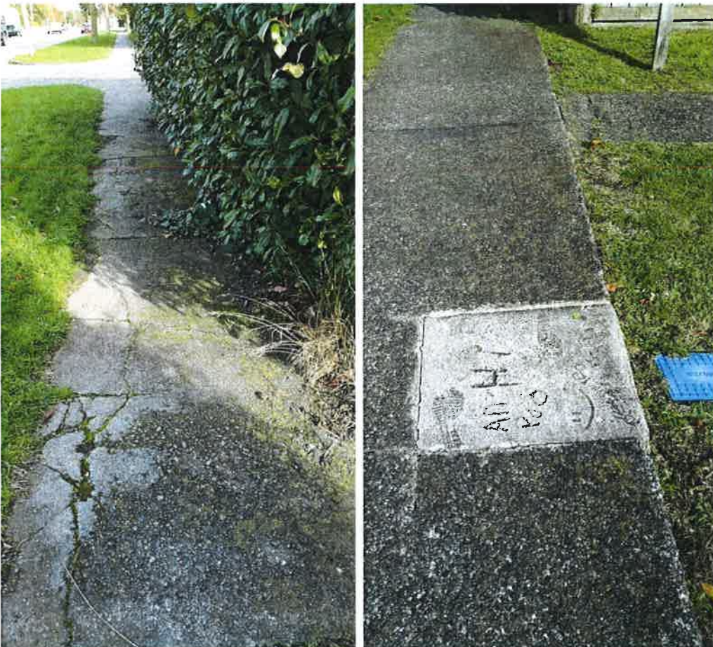
Repair with uneven surface
