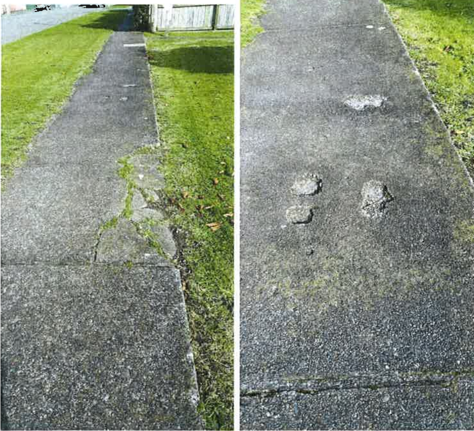
Hole in the pavement
